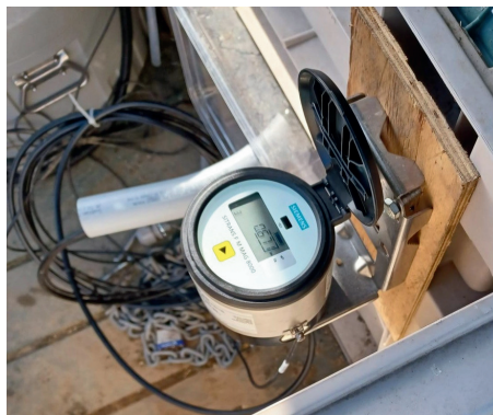
Magmeter installed in Tile A at Huronview (left); Rick Kootstra, Wim Feddes and Mari Veliz at Huron County Council (right).
