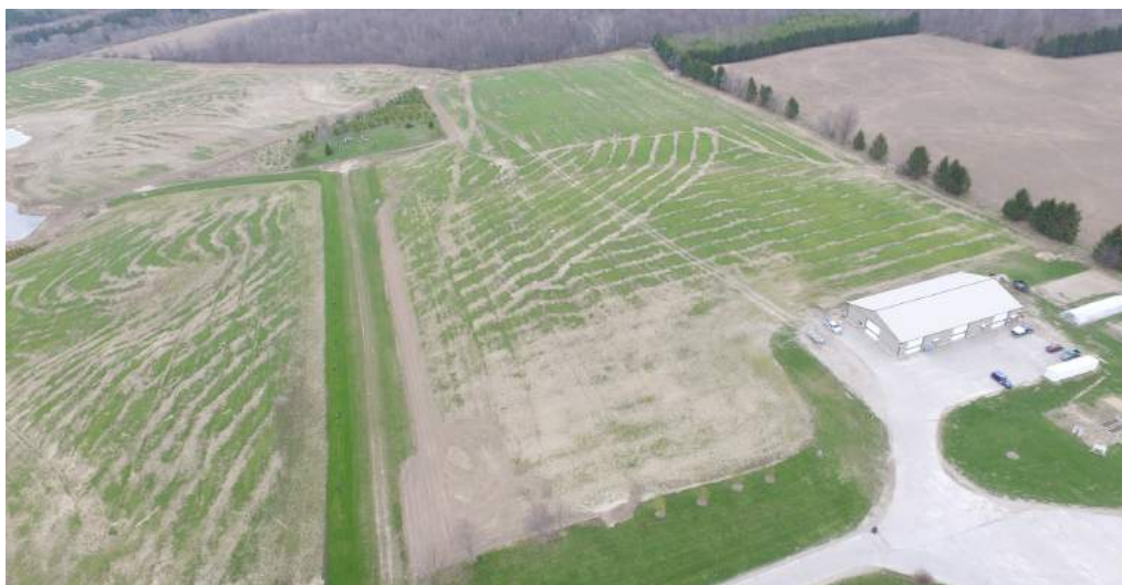
Aerial view of tile drainage after installation at Huronview.
